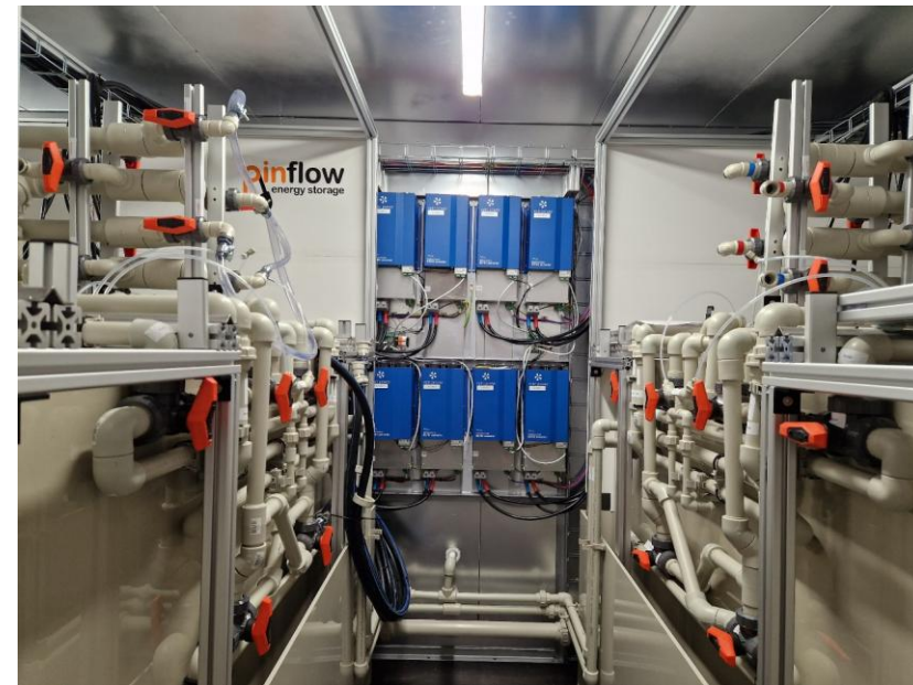
Pinflow – Czech Republic 100 kW – 250 kWh
