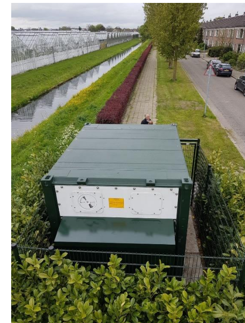
Rijsenhout: 140kWh/125kW Neighbourhood battery
