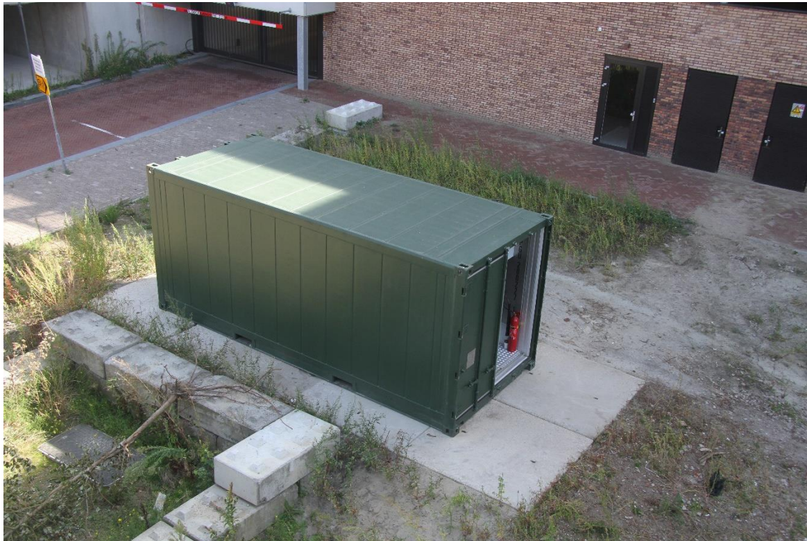
Eindhoven: 300kWh/350kW PV-energy storage and EV chargers
