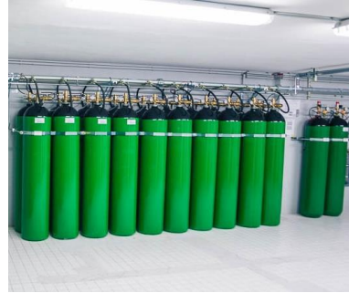
(residue-free) extinguishing with (Nitrogen) gaseous mixtures
