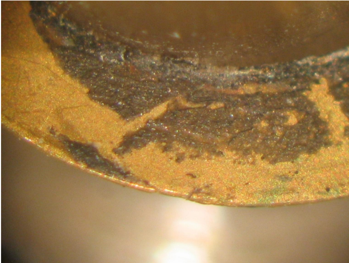
Corrosion products and other impurities on the contact surface (after 25 years of operation)
