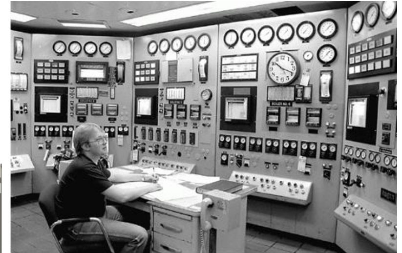
Boiler Operator Jeff Craigie sits in the Boiler Room and monitors flows, temperatures and pressures of the boilers and feed-water system. Photo by Ryan Solomon
