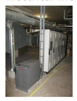
Custom built cabinets for power supply in Medical used rooms with Transformers, Impedance Monitoring, Visualization and UPS
